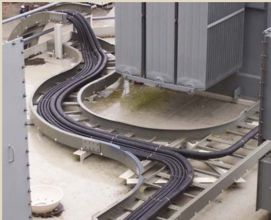
Crush and impact resistant CIR cable's smooth jacket, superior flexibility and lower overall installation costs make it the new favorite for oil and gas companies looking for innovative cable solutions.
